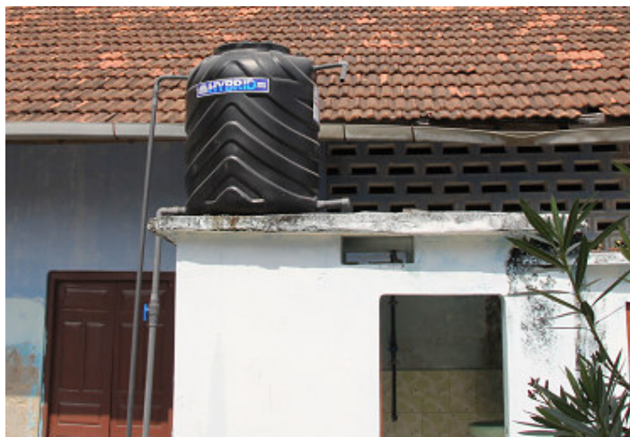
Feeder tank for drip irrigation system – Madya Maha Vidyalayam, Delft
