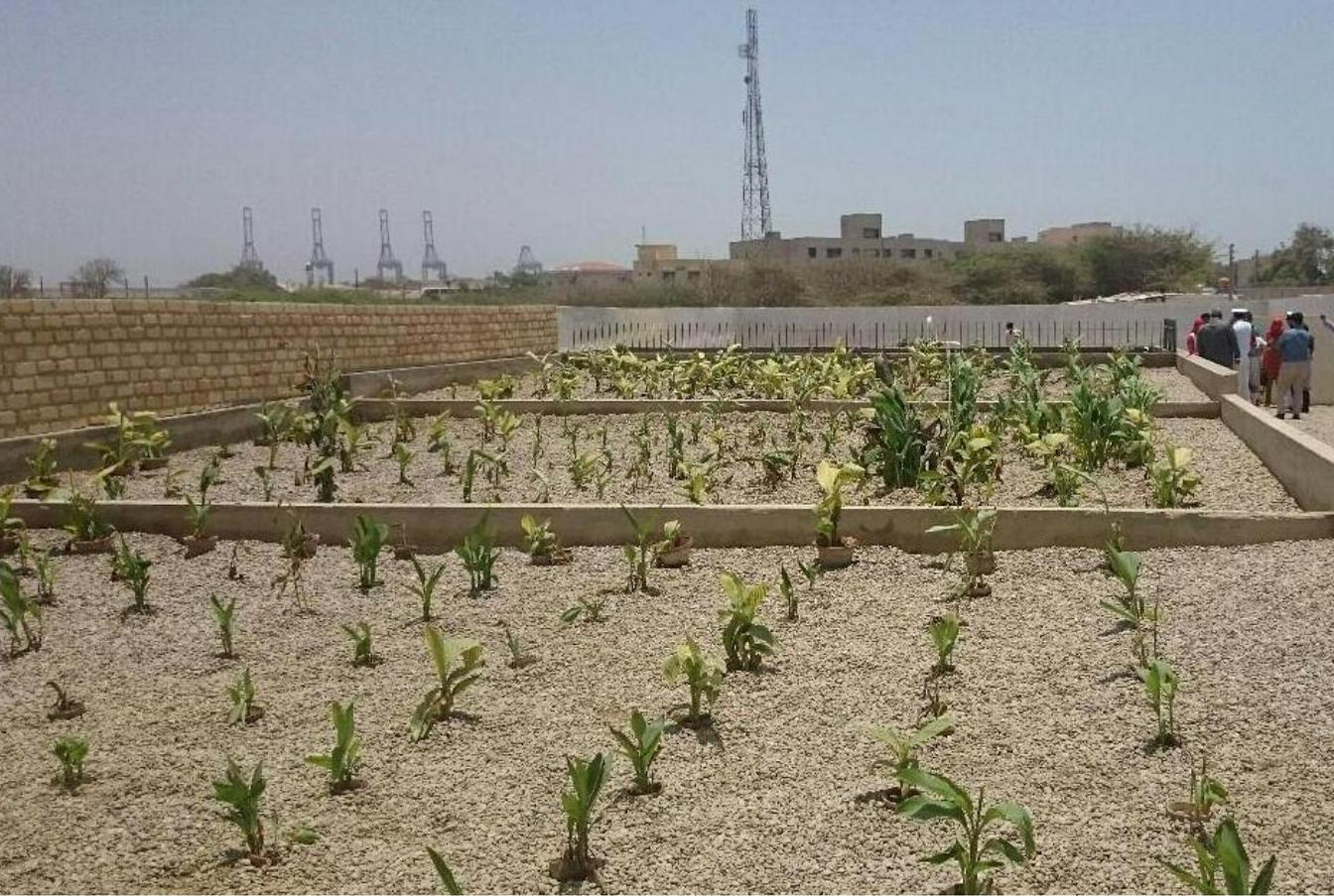
designed to imitate the processes found in natural wetland ecosystems. The system involves a series of gravel filter beds planted with reeds to treat wastewater passing through the root zone. The system is cost-effective as it is less energy-intensive than traditional wastewater treatment techniques and uses natural materials and processes. The project has helped in saving thousands of gallons of freshwater that may otherwise have been used for the greening purposes.
